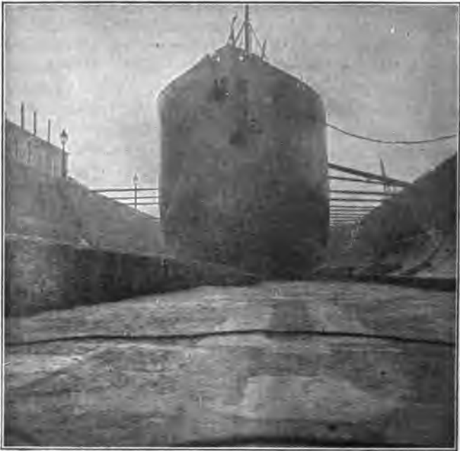
FIG. 287.—A tramp steamer in dry dock shows how nearly cubical she is—about 81 per cent.
